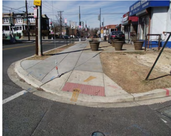
Figure 8 – Non-Standard Pedestrian Ramp
