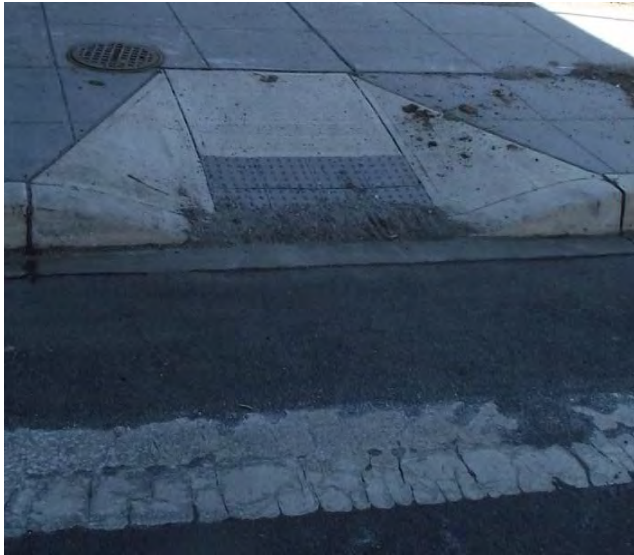
Figure 14 – Non-Standard Pedestrian Ramp
