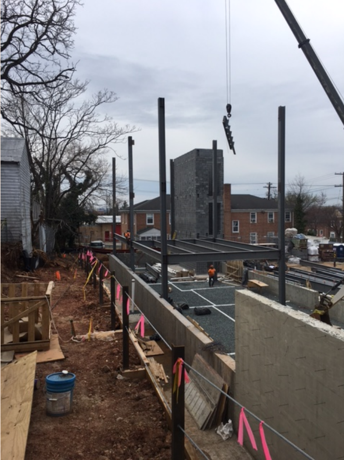
Structural Steel Installation
